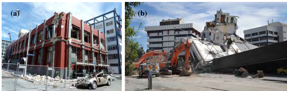
Figure 4. a) Two storeyed building with a reinforced concrete load bearing system. The ground floor is taller than the second floor. It seems to be quite robust and stiff. Its plan is orthogonal with the one dimension quite long. It seems as if it has been strengthened and probably the second storey has been added later. The
