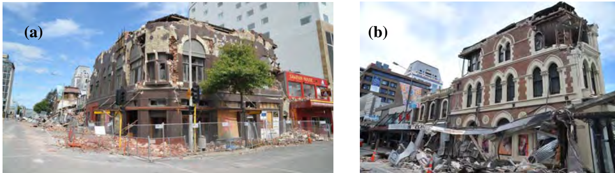
Figure 3. a) Three storeyed traditional corner building. It is an unreinforced masonry structure with higher storey heights. It is functioning as a shop in the CBD. Therefore the structure (floors and non load bearing structural members, the materials and workmanship) is strong enough. On the other hand the openings inside the building must be larger than common residential buildings. Nevertheless the facades present a robust structure. The vulnerability is estimated to be class C. The upper part and the corners of the building are damaged. It seems as if the roof had hammered over the lower part of the building. A large part of the roof collapsed. No horizontal displacements or diagonal cracks are noticeable. The observed pattern of damage is indicative of the strong vertical seismic component, a fundamental characteristic of the seismic action in epicentral regions of shallow focus earthquakes. The damage is grade 3 (substantial to heavy damage); b) Three storeyed unreinforced traditional masonry corner building. The building is functioning as a shop in CBD of the city. Each floor of the building is symmetrical along the two horizontal axes. There is also symmetry along the height. Also, it is quite well built, composing a robust structure. The plan of the building is trapezoidal having its shorter dimension perpendicularly to the facade. The stiffness along its shorter dimension is much smaller than along its facade. The vulnerability is estimated to be between class C and class D. The third storey suffered quite symmetric damage. The corner elements of the top, third, storey at the facade collapsed, while the roof is still standing up. Not any diagonal crack or any lateral displacement is noticeable. The only reason for the damage is due to the effects of the dominance of the vertical seismic motion. The damage grade is 4 (very heavy damage).
