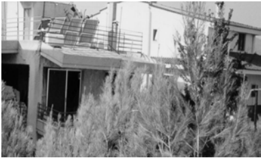
Figure 8: The cantilever slab dropped. Epicentral region, Parnitha earthquake, 1999.
