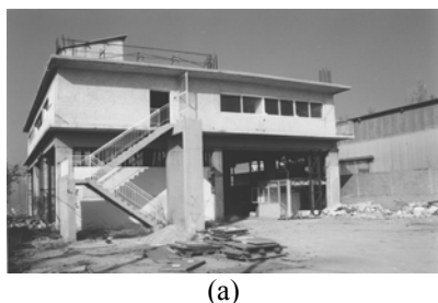
Figure 12: The books, bottles etc. on the selves have not been dislocated in the remaining part of the building, the other part of which was fully collapsed. The remaining part has brick walls down to the foundation. The collapsed part had no brick walls at the ground floor. Epicentral regions. fig (12a), Parnitha earthquake, 1999. fig (12b), Aegion earthquake, 1995.
