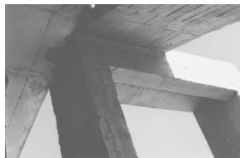
Figure 13: The staircase is statically independent from the rest of the structure with a gap of 2 - 3 cm. There is extremely small contact damage (due to horizontal motion) as shown in fig (13c). The whole building suffered extensive structural damages, as shown in fig (13b). Epicentral region, Parnitha earthquake, 1999.
