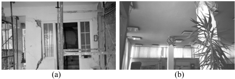
Figure 2: There are no damages justifying important horizontal motion. Notice that the windows are unbroken in both cases. Explosive type of damage. fig (2a): Epicentral region, Parnitha earthquake, 1999, fig (2b): Epicentral region, Aegion earthquake, 1995.
