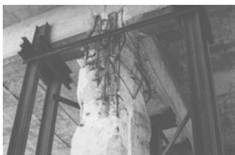
Figure 13: The staircase is statically independent from the rest of the structure with a gap of 2 - 3 cm. There is extremely small contact damage (due to horizontal motion) as shown in fig (13c). The whole building suffered extensive structural damages, as shown in fig (13b). Epicentral region, Parnitha earthquake, 1999.
