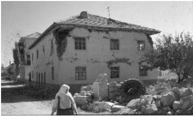
Figure 3: It is evident the vertical action during the Dinar, Turkey 1995 earthquake (no diagonal cracks). Symmetrical damages around a vertical axis of symmetry, horizontal cracks on the first and second levels.
