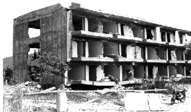
Figure 16: Ground floor collapse. The hypocentre is close to the foundation of the building. Epicentre of the Rio, near Patras earthquake M=4.2 , 1974.
