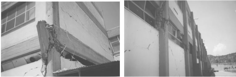
Figure 15: The damaged columns are not due to the 'short column' case. The damages are transverse to the plane of the brick walls. Note that the windows are unbroken. Epicentral region, Aegion earthquake, 1995.
