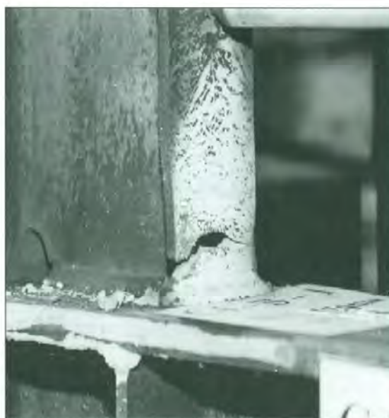
Fig. 7 Typical failure mode, with weld cracking.
