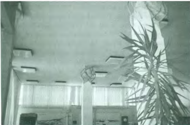
1a – Eagio (1996) earthquake. The crushing of concrete and the symmetrical buckling of bars are apparent. The vertical edges of columns are still aligned.
