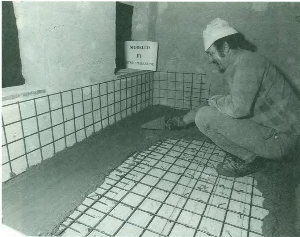
Figure 5. Steel network and cement layer over the slabs (sn)
