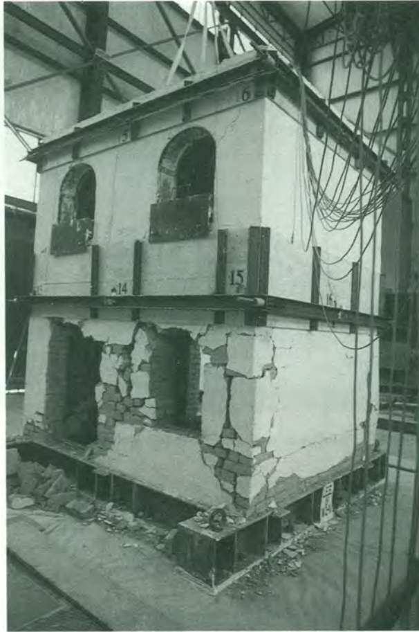
Figure 7. Building M2, strengthened by wp-ht-hb-a2, after the last shock
