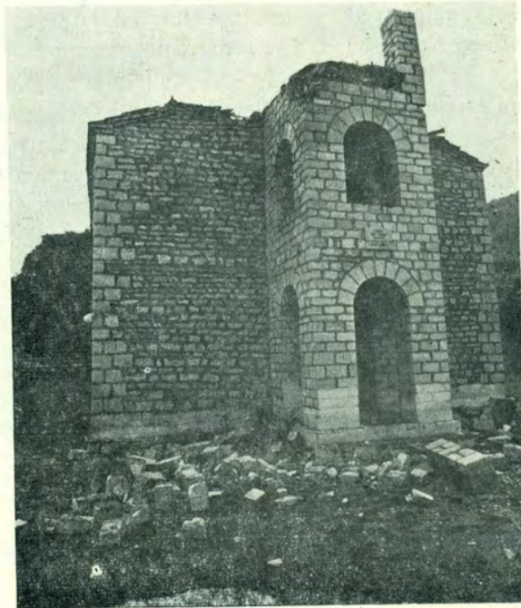
Fig. 34. The steeple was struck by the main body of the church at Kaloudi, giving also a rotation to its top part, after the first earthquake (a). The third earthquake caused the overturning of the top part of the steeple, which fall into the church (b).
