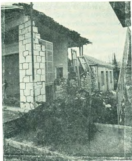
Fig. 22. Old house half collapsed after the third earthquake (b). It was not repaired after the first earthquake (a).
