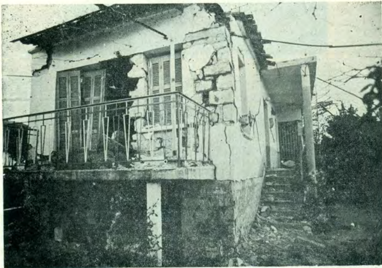
Fig. 32. Destruction of a contemporary one and a half story building after the third (b) earthquake, while it was not repaired after the first one (a). The destruction of the front parts of the wall is proportional to their rigidity.
